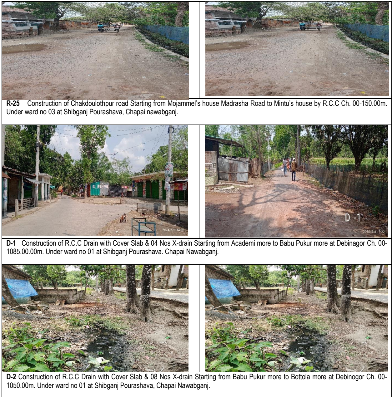
Figure 4: Existing Road and Drains Picture
